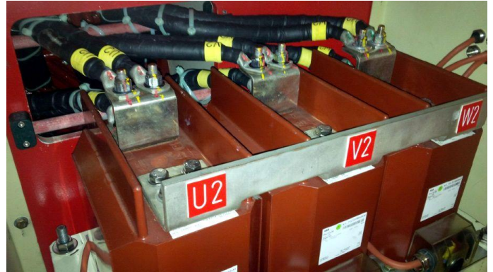
Neutral point with neutral point converter
