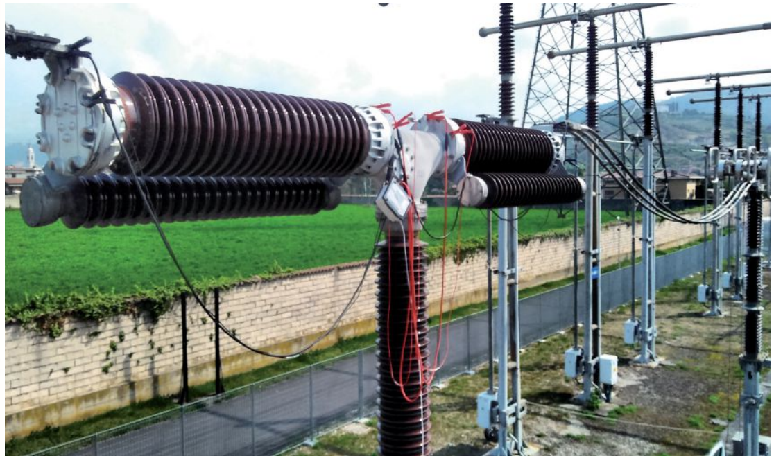
Measuring Setup in the Field
